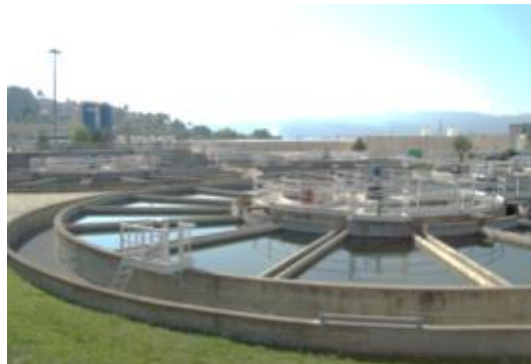
Waste Water Treatment
