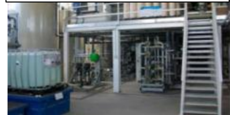
Municipal Reclaim System
